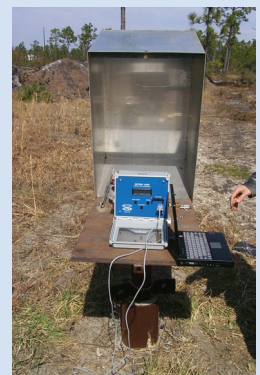
Sutron 8400 recorder installation with laptop for data download. (Photograph by Bill Cunningham, USGS)
