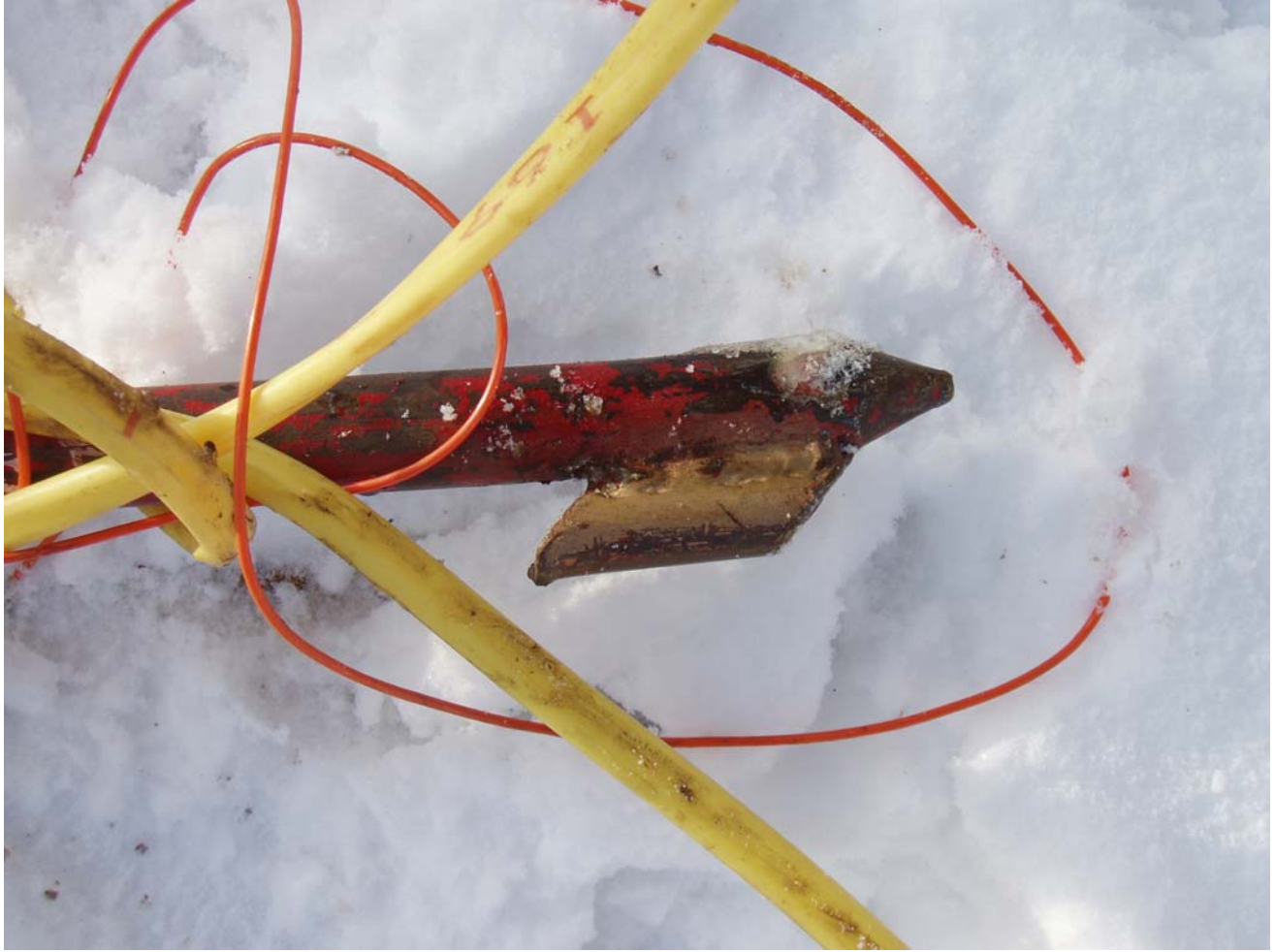
Figure 2.1-3 Tip of fishing tool at R-33 with retrieved Barcad tubing
