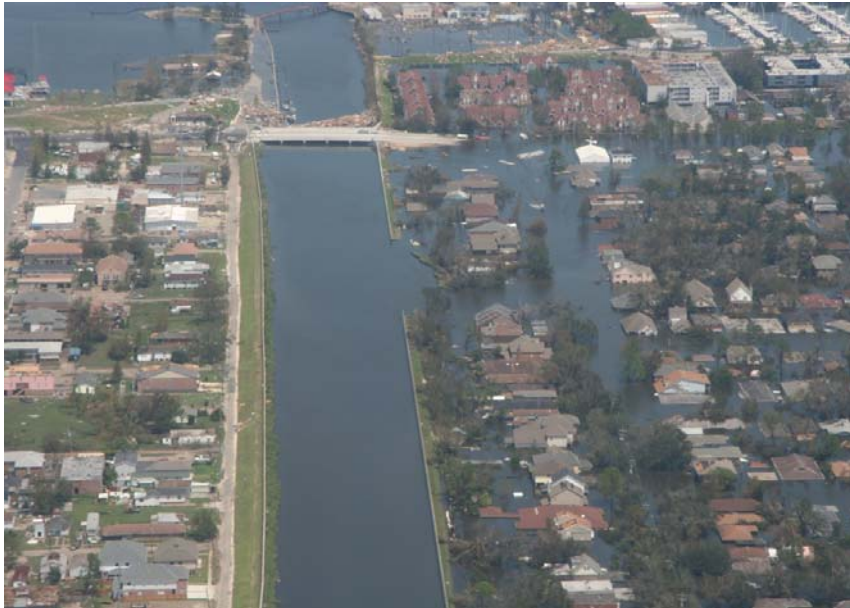
17 th Street Levee Breach
