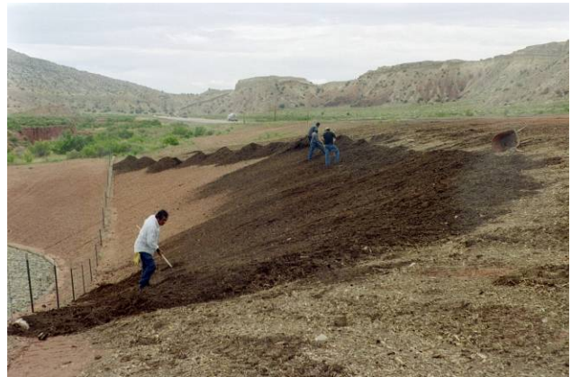
San Ysidro, NM - Highway 550 NMDOT seeding trial. Spreading mulch on construction slopes.
