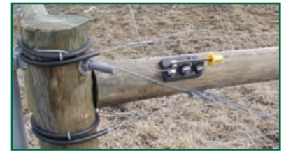
Cut-off switches are handy because they allow you to turn off sections of the fence for repairs and to locate shorts.
