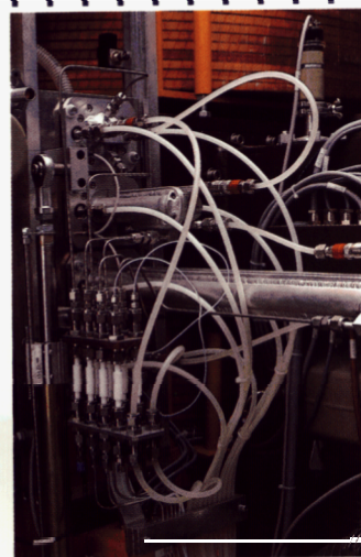
The most common method of producing radiopharmaceuticals is with a cyclotron installed in the medical center basement. Shown are a typical cyclotron and the targets utilized to produce the short-lived positron emitting radio-nuclides.
