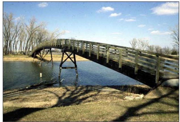
Figure 5—Yellow-cedar is durable and suitable for structural applications.
