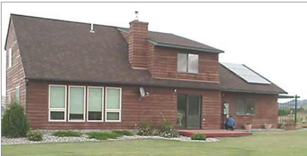
Net-metering helps make grid-tied photovoltaic systems more economical. This home in Bozeman gets some of its power from a 1-kilowatt PV system that is tied to the utility grid.
