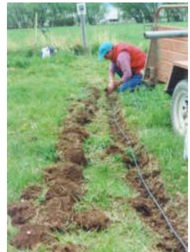
Burying cable in a shallow trench. (NCAT photo)
