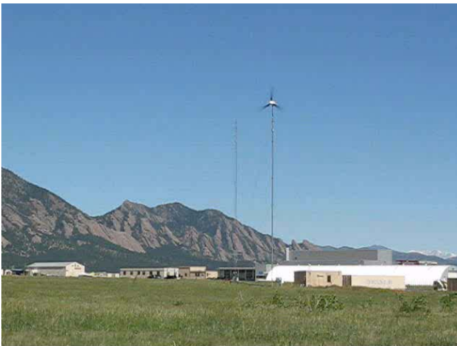
Figure 11. Infrastructure Upgrades for Small Turbine Independent Testing
