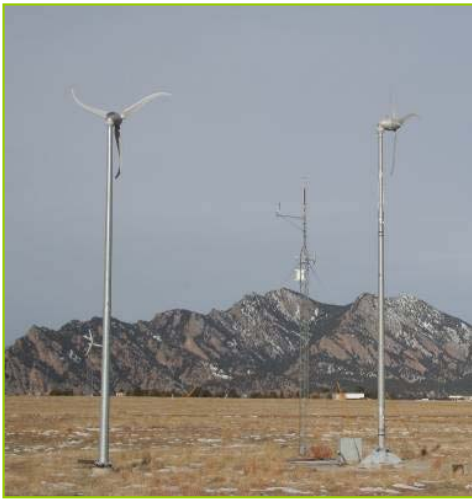
Figure 12. Skystream 3.7 wind turbines
