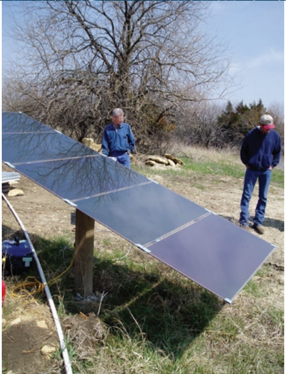
Solar pumping systems move water to alternative watering systems in the Marais des Cygnes River Watershed in Kansas. The Franklin County Conservation District and partners are working to help producers install watering systems and protect fragile streams.
