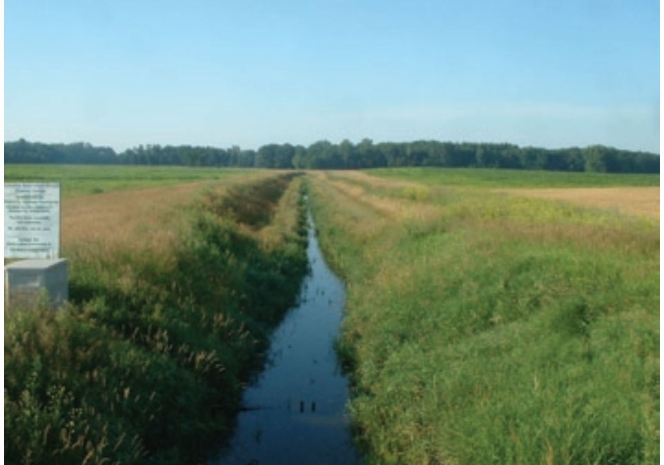
A naturalized stream channel design for an Ohio drainage ditch incorporates “benches” and vegetative filters. Sponsors of the model project included Mr. and Mrs. Joe St. John, Hillsdale Soil and Water Conservation District, Hillsdale County, the Hillsdale County Drainage Commission, NRCS and Ohio State University. Funders were The Nature Conservancy and the Great Lakes Commission.
