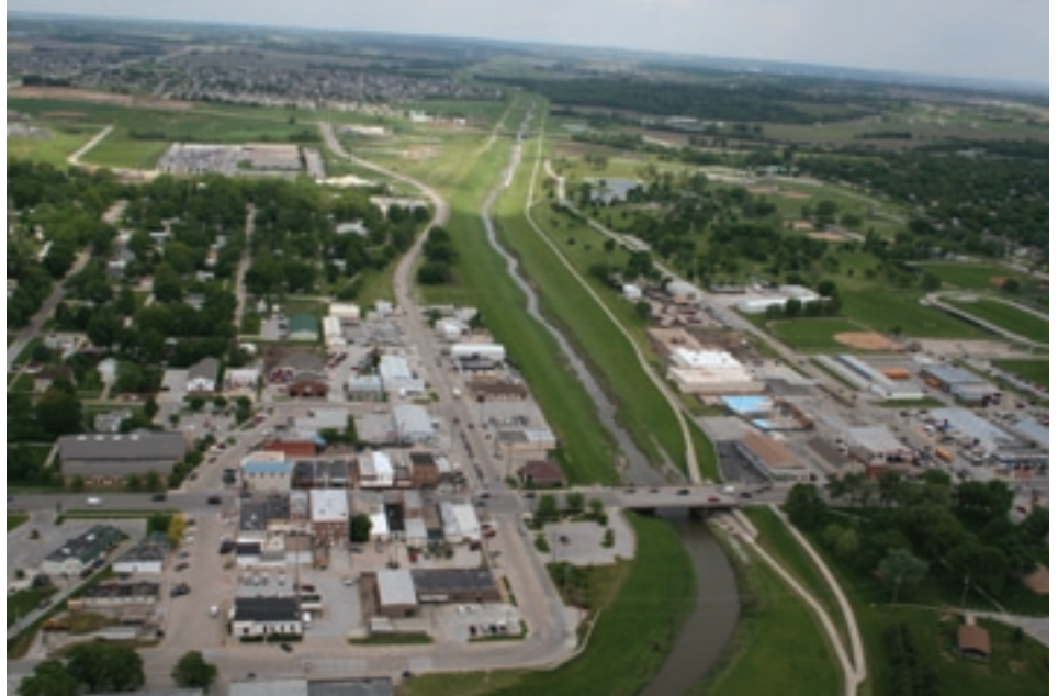
A drainage and flood control channel in the community of Papillion is lined with trails that people use for walking, biking and other activities.
