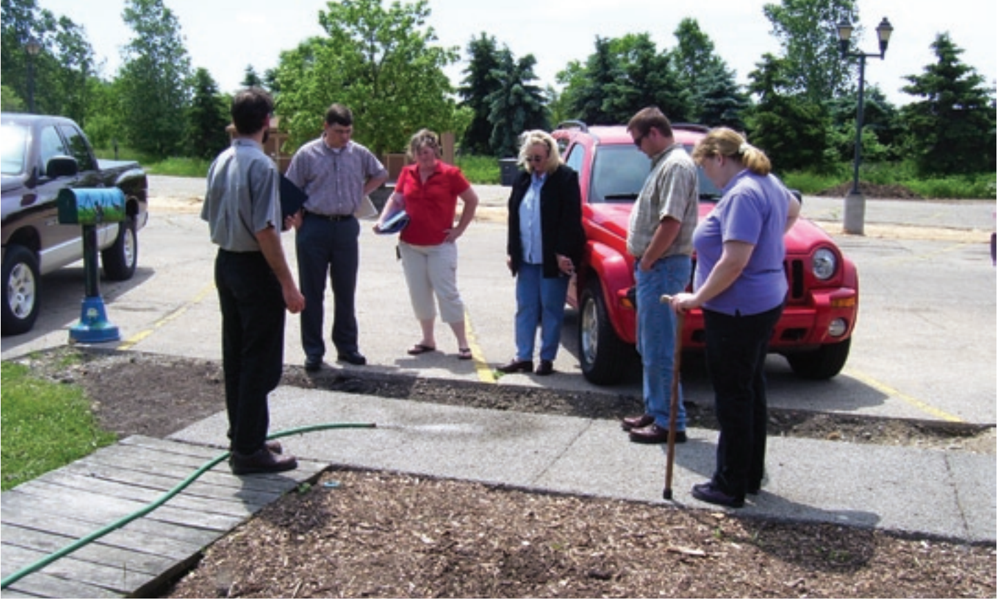
Permeable pavement at the city of Elkhart Environmental Center increases on-site storm water infiltration. It is among many practices recommended by the Elkhart River Alliance.
