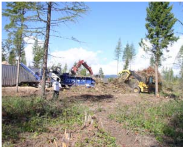
Figure 28—Loader on right of photo used to retrieve loose material from nearby slash piles and feed material to the excavator. (Bonners Ferry, Idaho, 2006).
