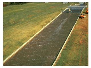
Research into the use of vegetation for erosion protection has allowed extensive use of vegetated earth emergency spillways on flood control dams. When suitable, these spillways offer both aesthetic and economic advantages over conventional structural spillways.
