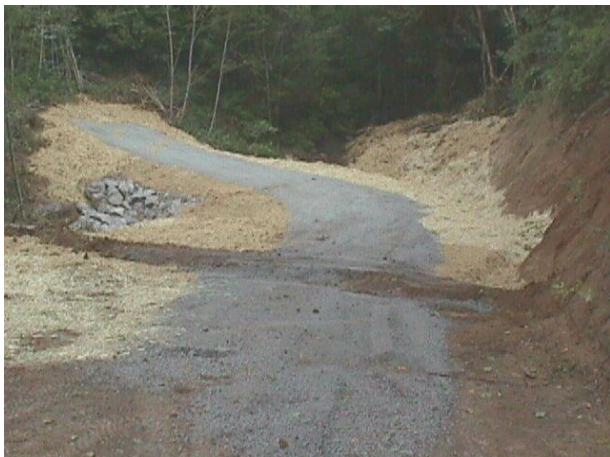
Seeding and mulching at a culvert replacement site
