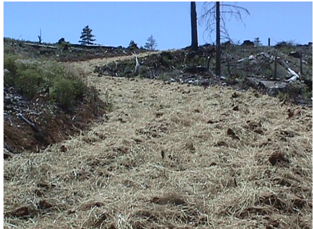
A road decommissioned by ripping, mulching, and seeding
