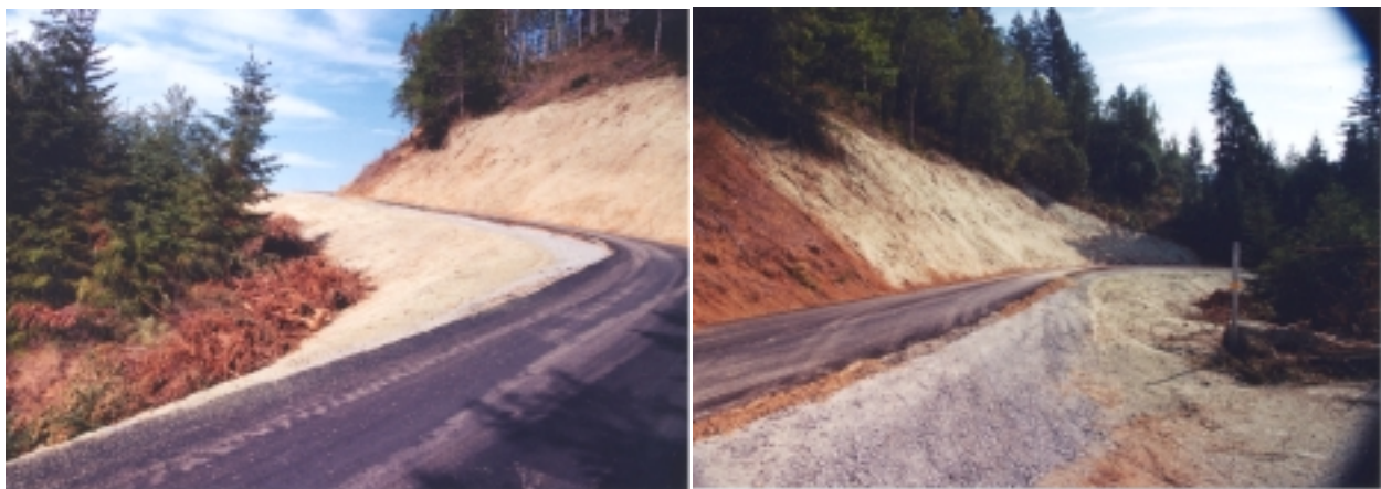
A portion of the ERFO repair on the Elk Mountain Loop Road.
