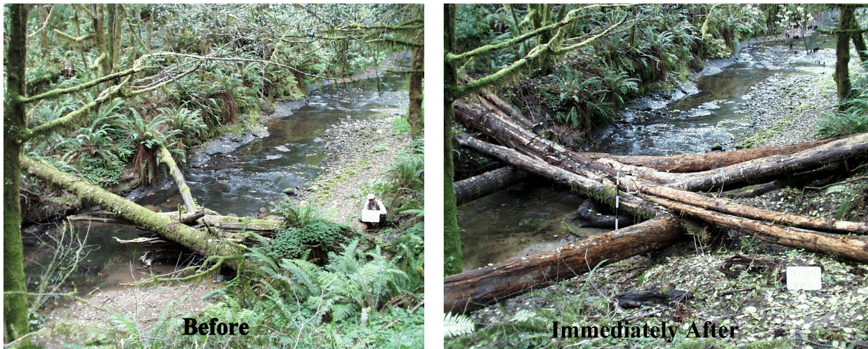
Figure 3. An example of before (1999) and after (2000) channel cross section data for the South Fork Elk Creek in-stream restoration project. Notice that there has been substantial gravel deposition as a result of
