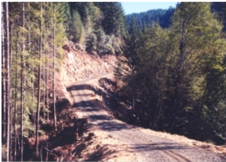
Road constructed under Right-of-Way Agreement in the Tioga Creek area.
