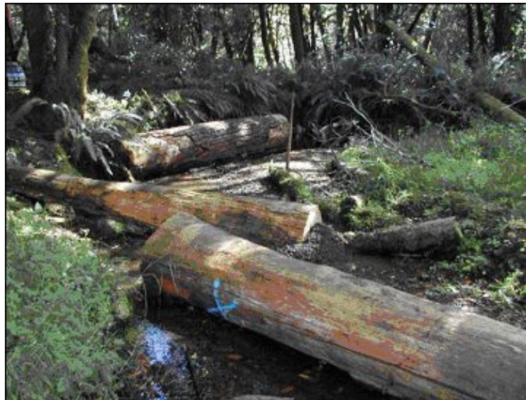
Blue Creek Instream Restoration Project
