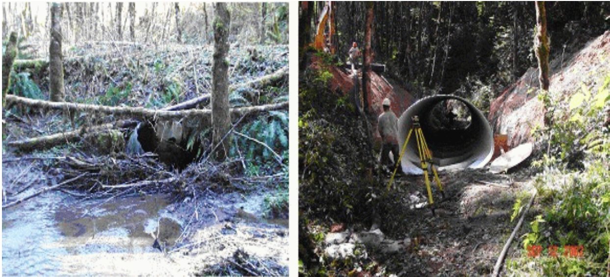
Right Fork Yankee Run Creek before and during culvert replacement
