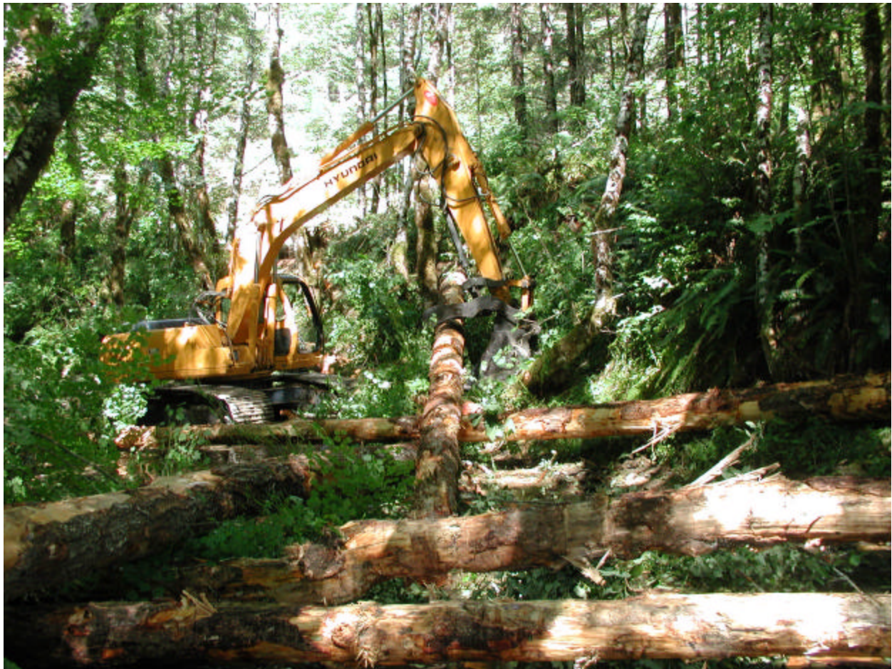
Local contractor using excavator to place wood in Big Creek.
