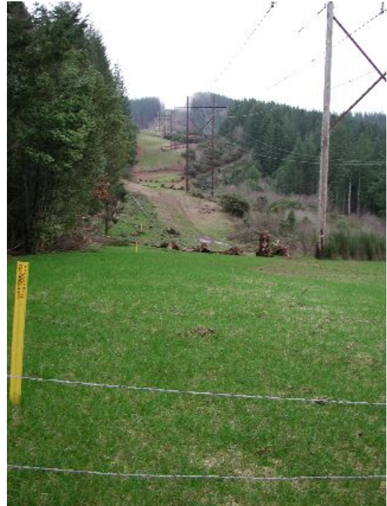
Natural Gas Pipeline Project - post construction – showing Erosion Control Stabilization
