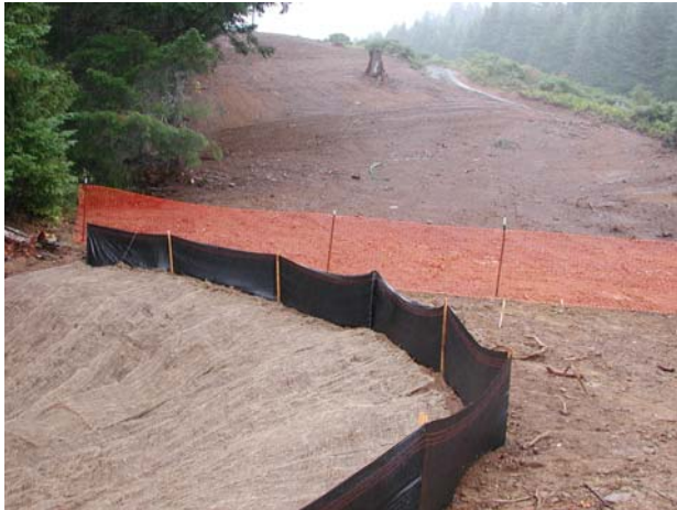
Coos County Pipeline project -during reconstruction
