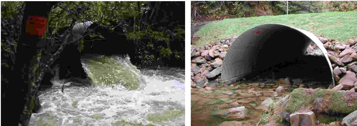
Figure 3. China Creek culvert before and immediately after replacement.
