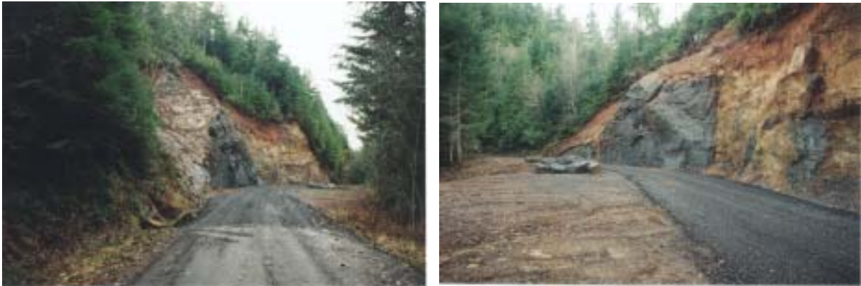
A portion of the North Fork Ridge Road repair project.
