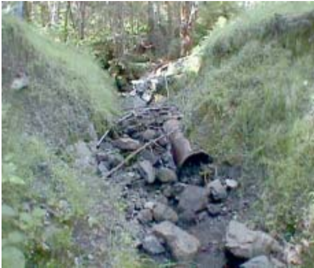
Stream Channel before reconstruction efforts
