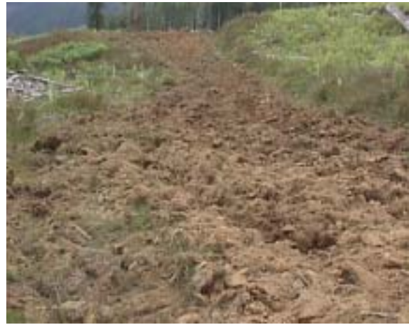
Final result of road surface after sub-soiling, a plantable surface
