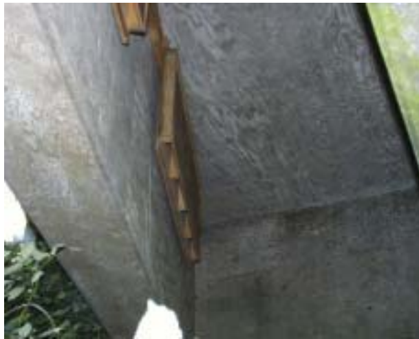
A small bat box retrofitted to a bridge
