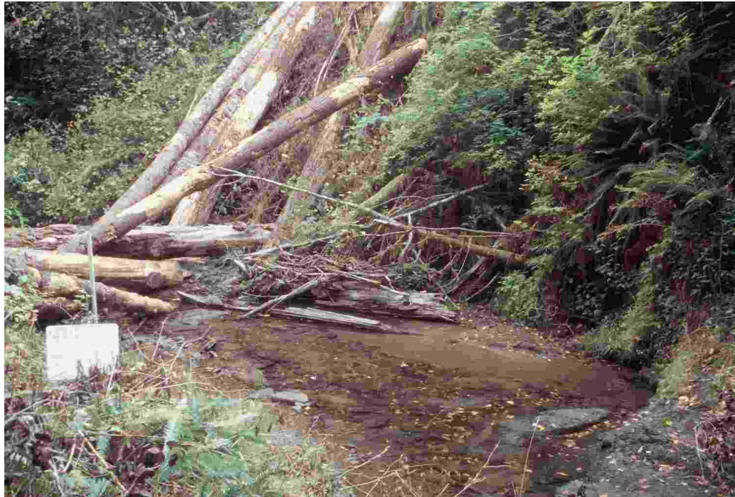
Figure 5. Recently placed logjam structure in Steel Creek
