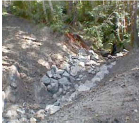
Channel widened and protected from stream velocities
