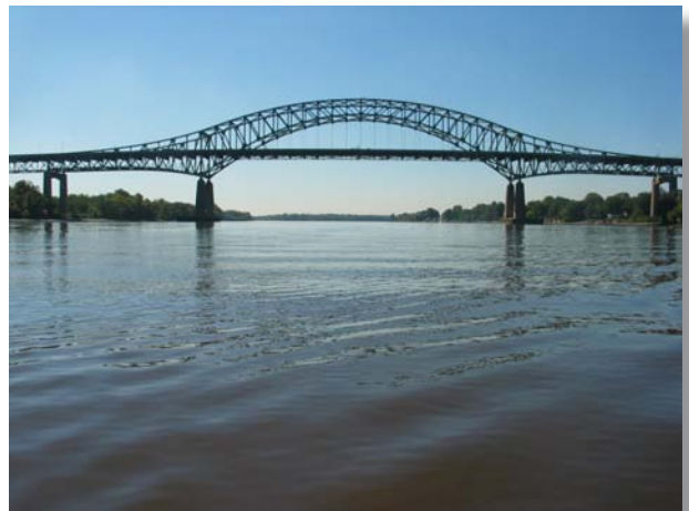
The Delaware River Bridge
