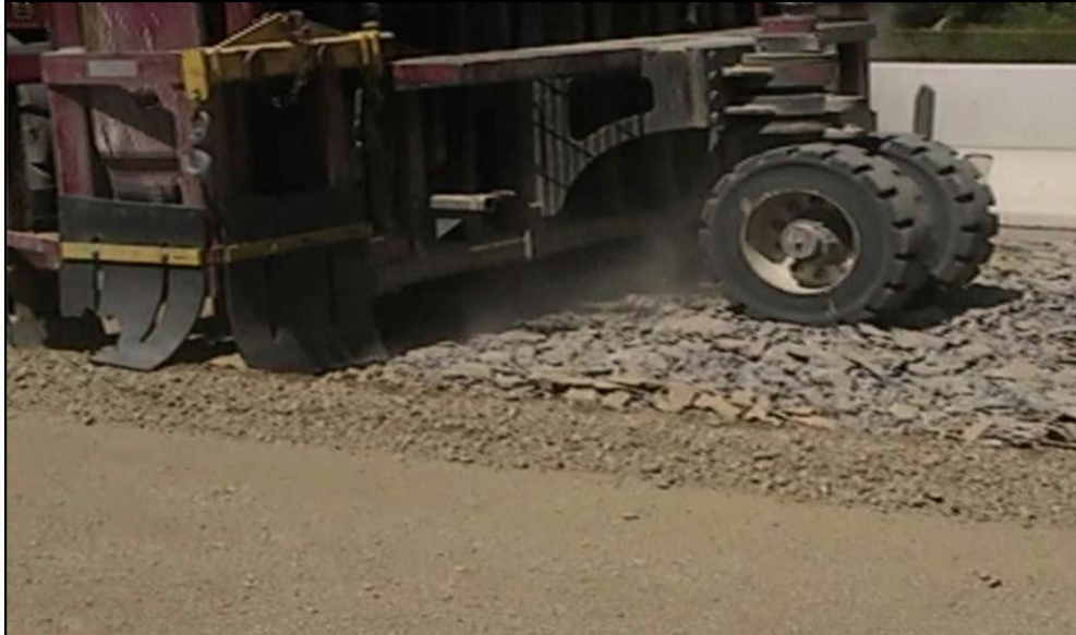
I-295 Concrete Rubblization Project
