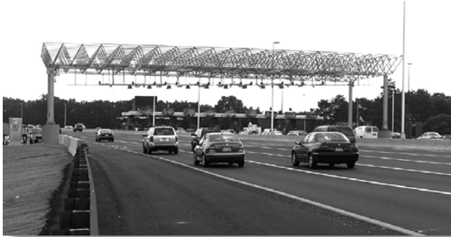
Express E-ZPass Gantry
