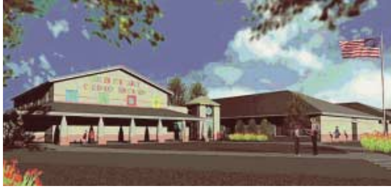
The New Early Childhood Center No. 45 in Elizabeth was built with funding from the state's $8.6 billion school construction program. It provides 20 preschool classrooms for 300 three- and four-year-olds.
