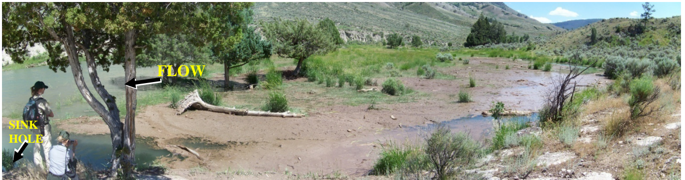
FIGURE 22: Photograph of Gardner River upstream from DFA. Note the ponding of the Gardner River caused by the constriction of the river channel. Water level is raised about 1.5ft. Brown area is organic matter floating on water surface. Sink hole cannot be seen from photograph, arrow points to general location, see Map 2 for regional location. Photograph taken 25 July, facing east.
