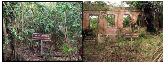
Figure 54: America Hill Project, Virgin Islands NP, before and after treatment.
