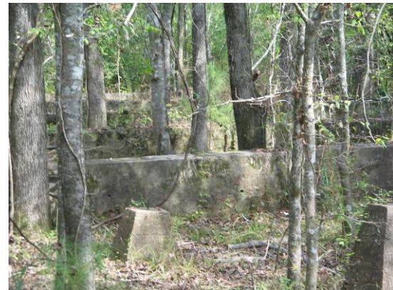
Figure 34: The 20.5 acre Voht Mill site was obscured by an understory of Chinese privet that has been removed revealing building structural features and artifacts.
