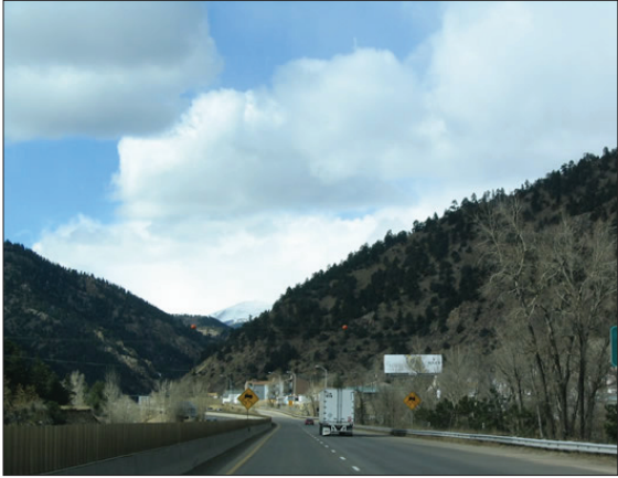
View of Interstate 70 approaching Idaho Springs. The Section 106 case regarding development of the transportation corridor associated with the interstate west of Denver is now closed.
