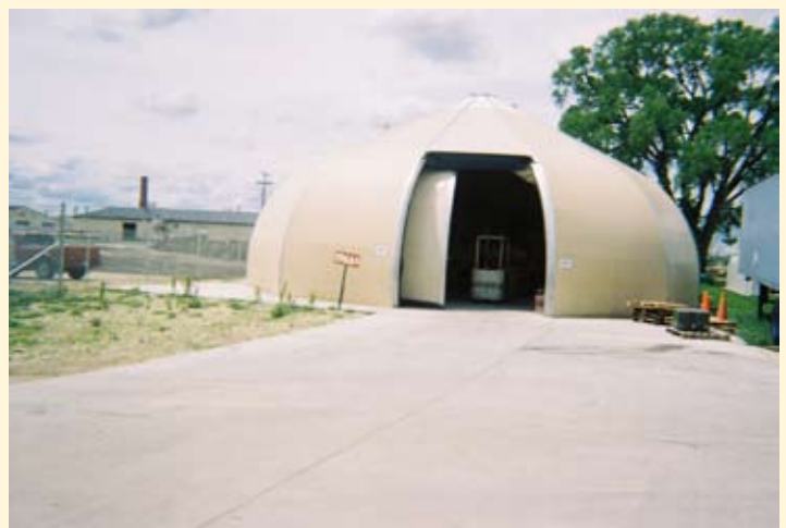
AAA relocatable building at Fort Riley.
