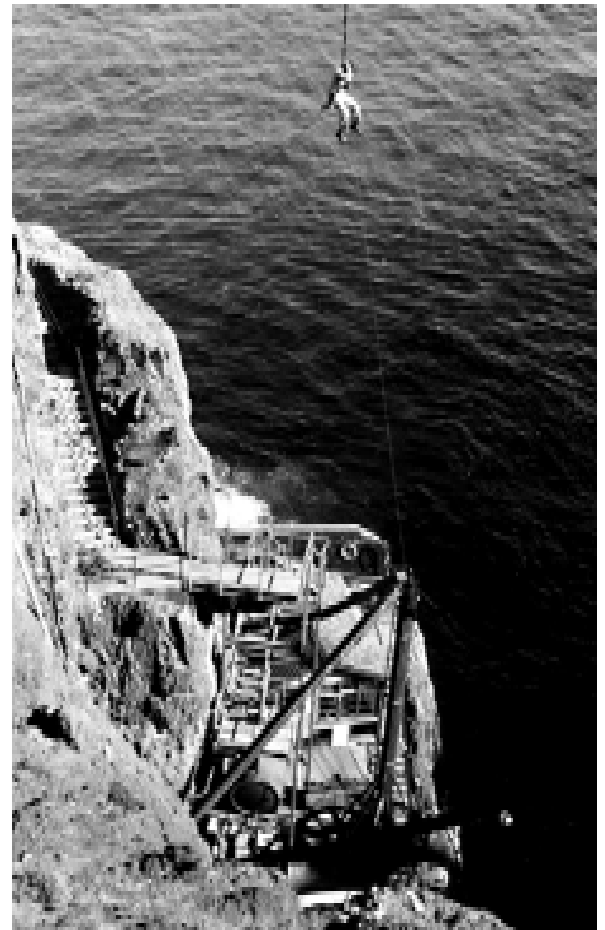
▲ Figure 2. Unconventional means were sometimes used to determine elevations. Here a coast surveyor keeps a tape vertical while being hoisted by a U.S. Coast Guard crane at Anacapa Island, California.
