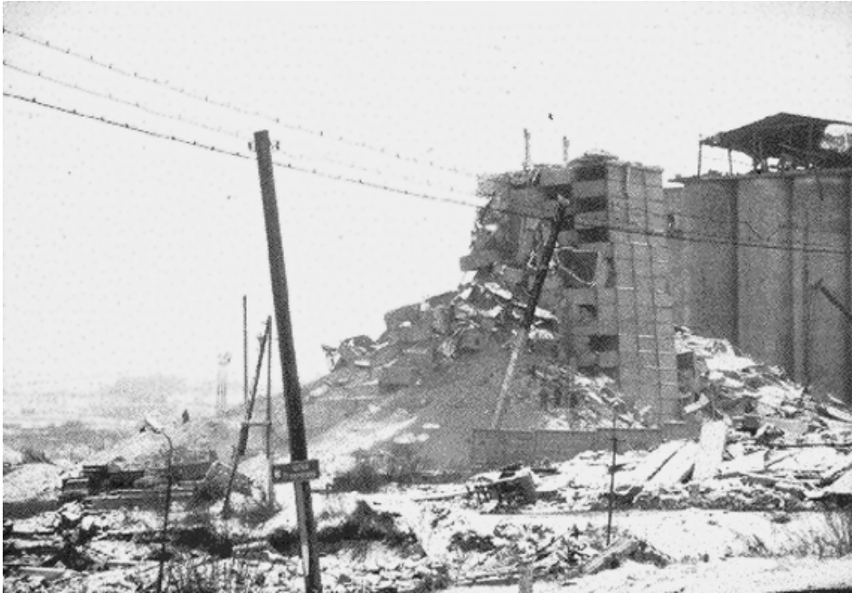
▲ Granary in a flour mill complex east of Spitak (grain can be seen spilling out of the collapsed concrete shear-wall structures in the foreground). This image from the Spitak Earthquake CD-ROM is available for viewing online through the WWW.
