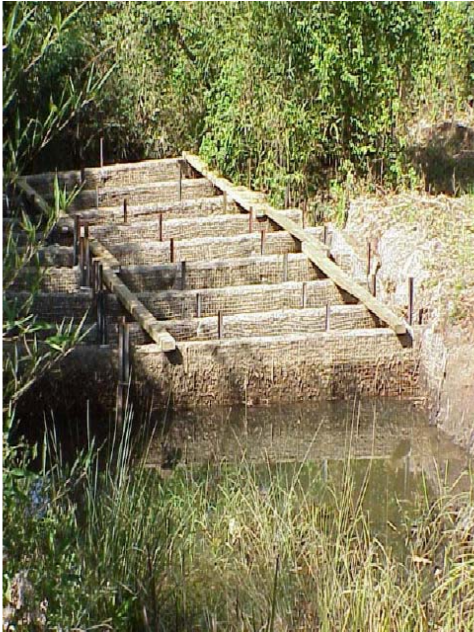
Figure F-4. Baffle grids used for filtering treated stormwaters (Iwinski, 2004).
