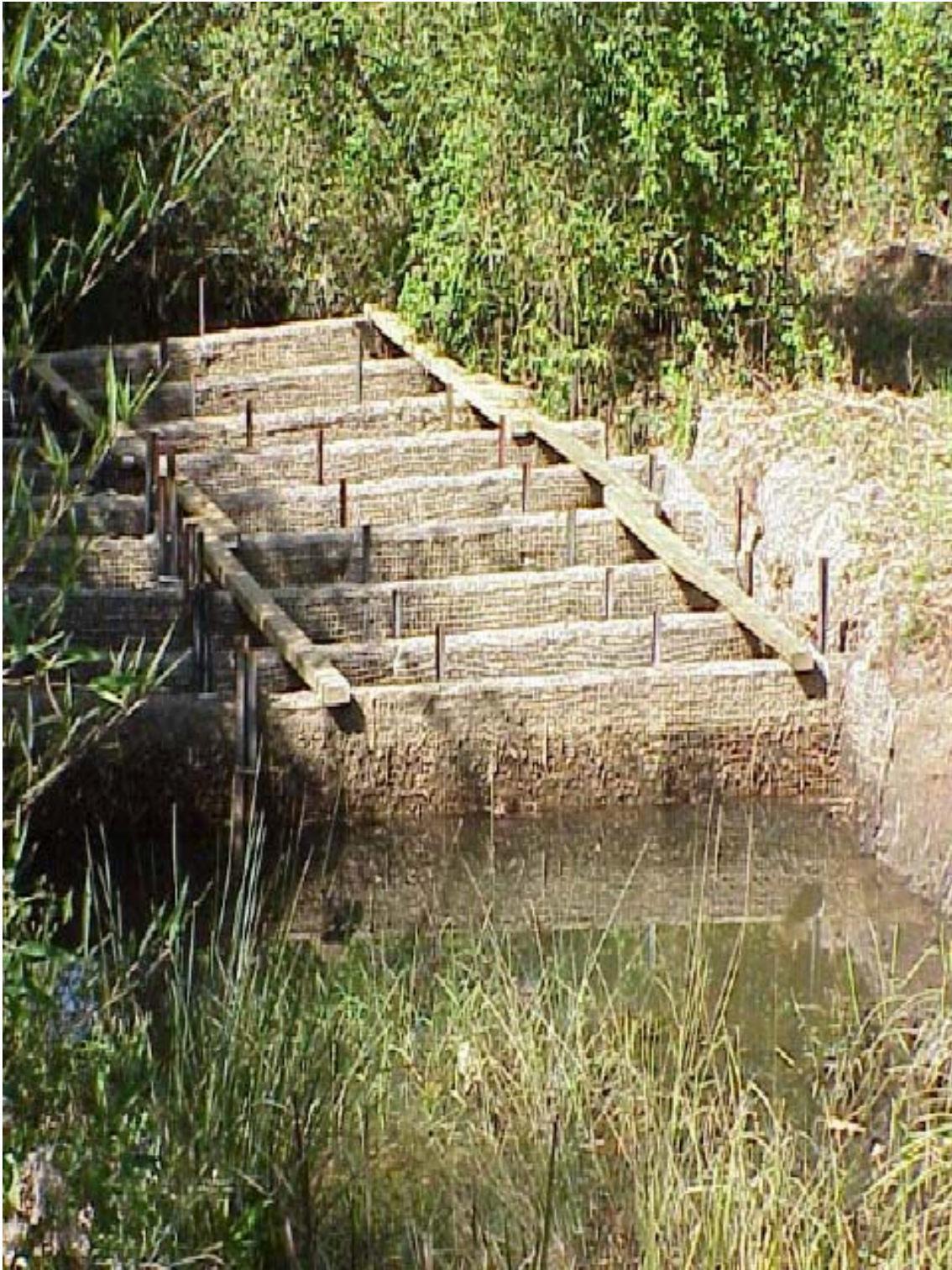
Figure 4 - 2. Baffle grids used for filtering treated stormwaters (Iwinski, 2004).
