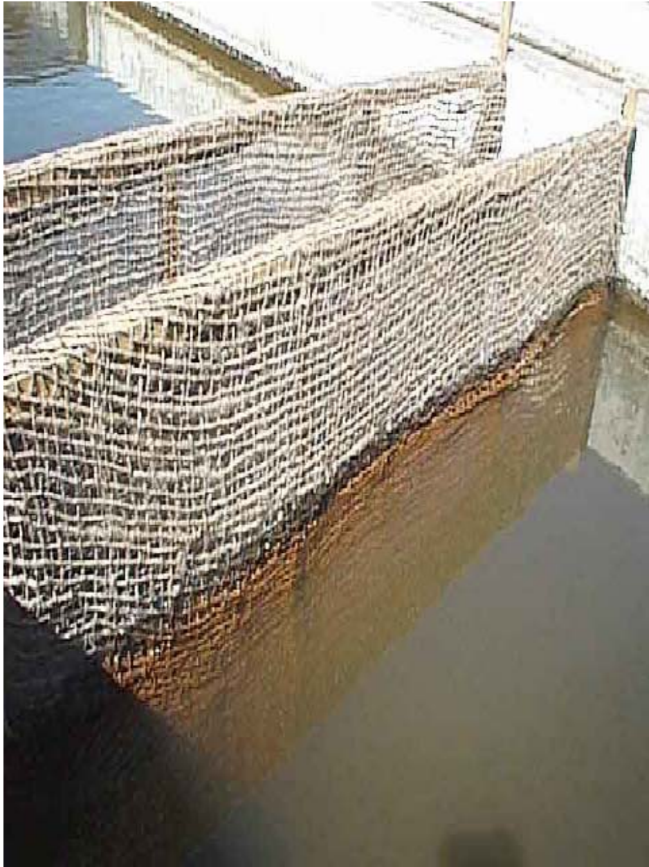
Figure F-3. Particle curtains of woven jute on wood frames (Iwinski, 2004).
