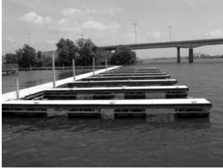
BIG Tier II project with transient boat slips/docks and piers.
