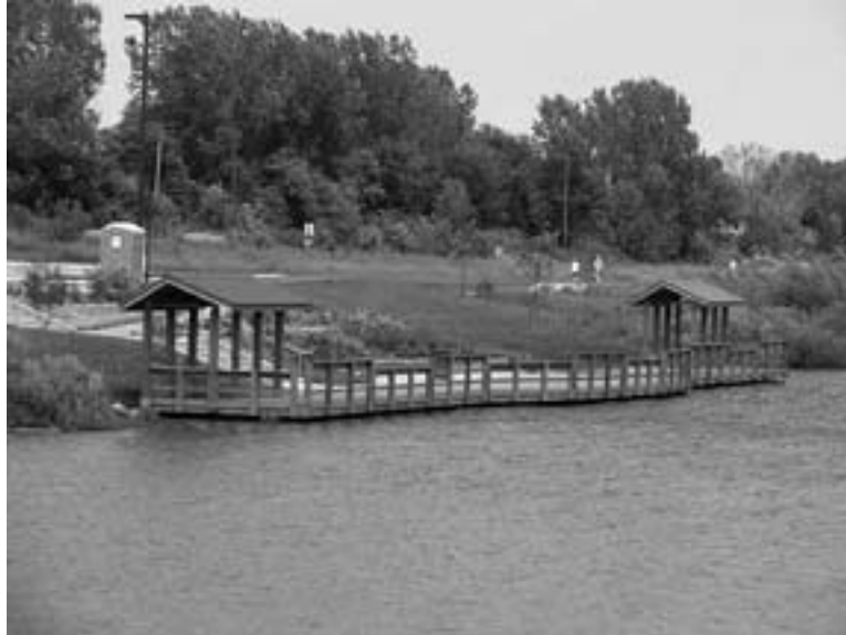
Blue Heron Fishing Pier, a partnership project with the City of West Des Moines on an urban lake in Iowa.
