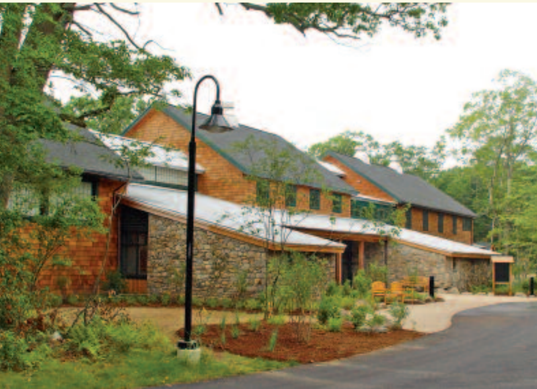
Red cedar shingles and local stone add texture to tradition in the new, energy efficient Rhode Island NWR Headquarters. (Janis Nepshinsky/USFWS)
