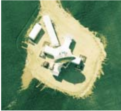
Doppler radar installation.
