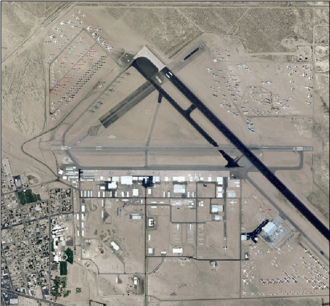
Figure 3-16. Aerial View of Mojave Airport
