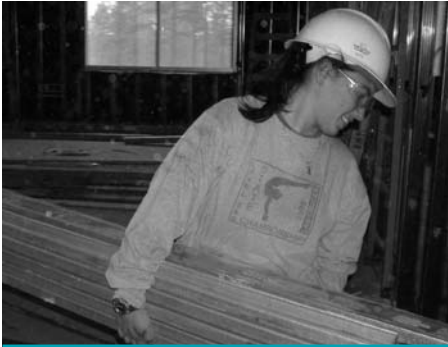
Kari Chung works as an apprentice on the EOC building.
