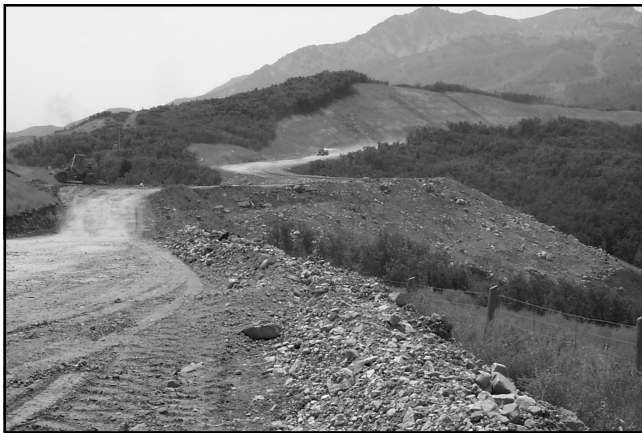
Snowbasin Connector road construction.
