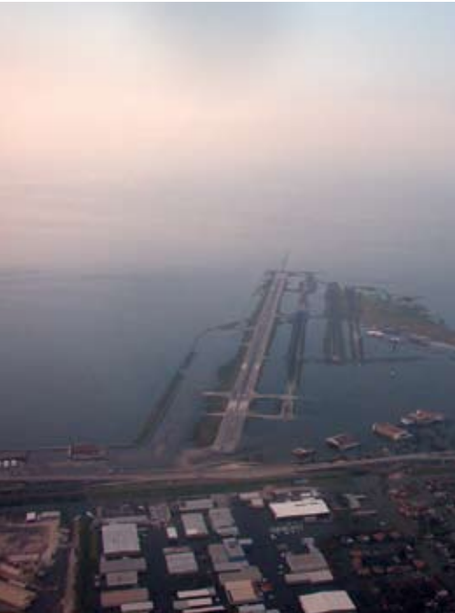
Flooding from hurricane Katrina covers the runways at the New Orleans airport. The FAA reopened a runway at this airport within 24 hours, making it possible to bring in life-saving supplies and evacuate people. Photo: FAA
