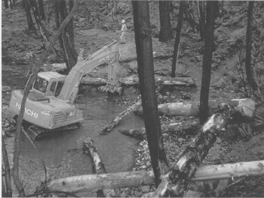
Figure 28: Heavy Equipment Working in Stream
