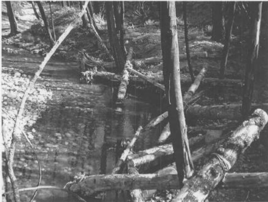
Figure 29: Completed placement of woody debris in stream
