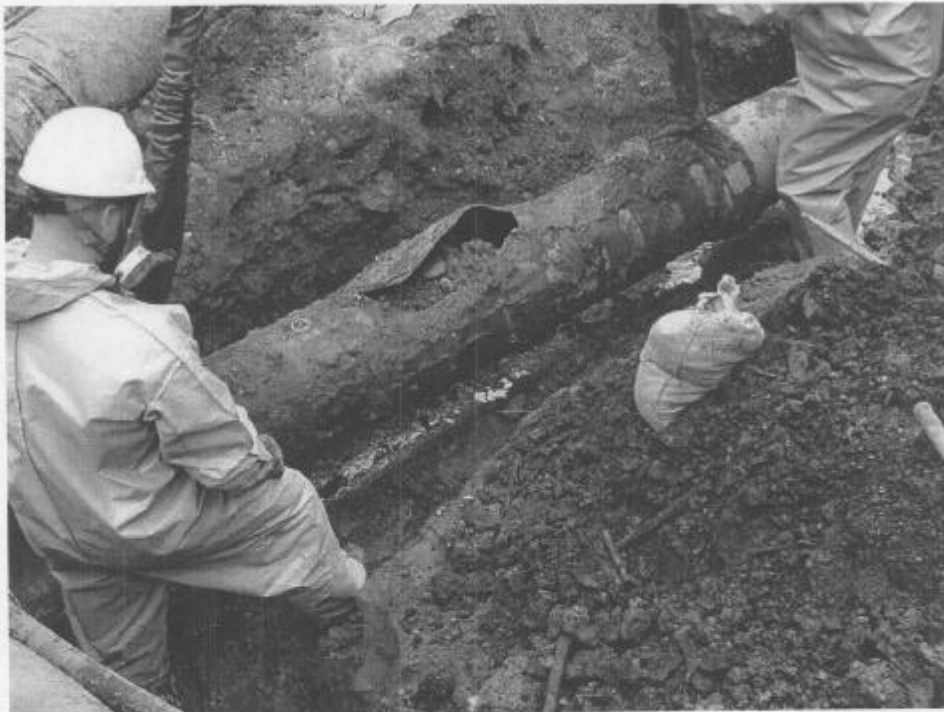
Figure 3: Excavation of Pipe
