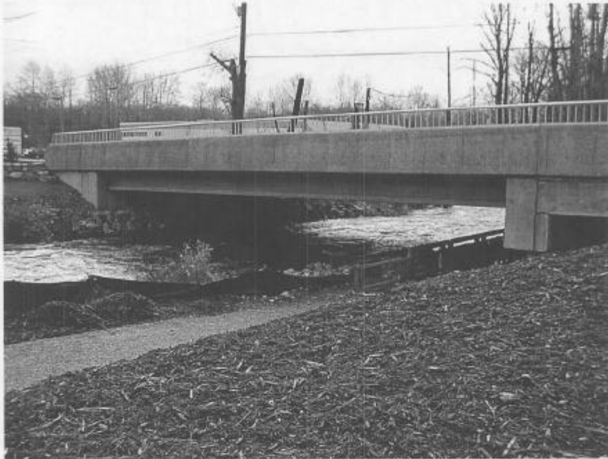
Figure 36: New Valencia Street Bridge
