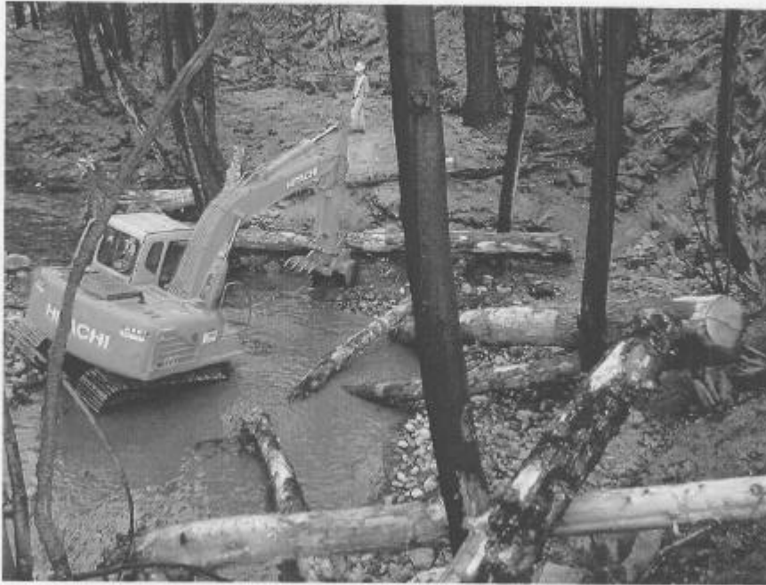
Figure 28: Heavy Equipment Working in Stream
