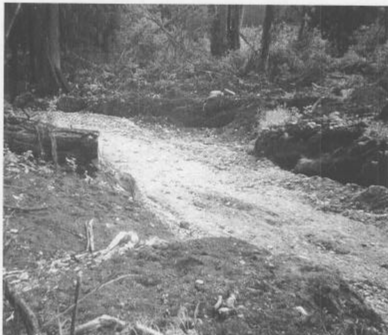
Figure 19: Hanna Creek Remediation (Before)
