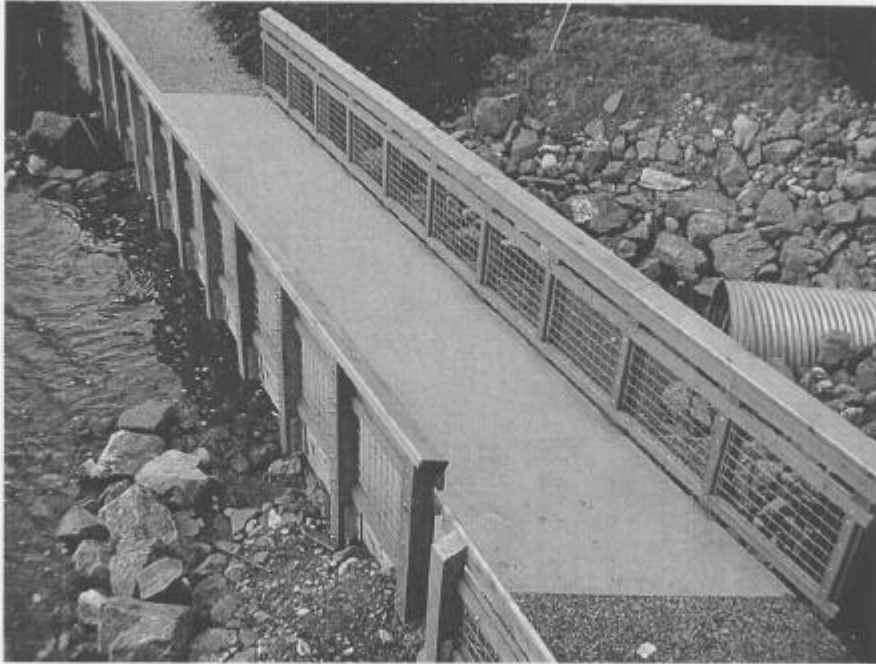
Figure 35: New Fever Creek Bridge
