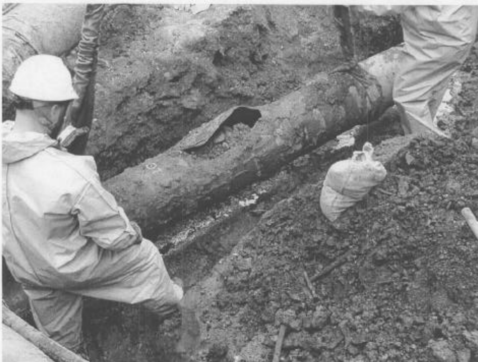
Figure 3: Excavation of Pipe
