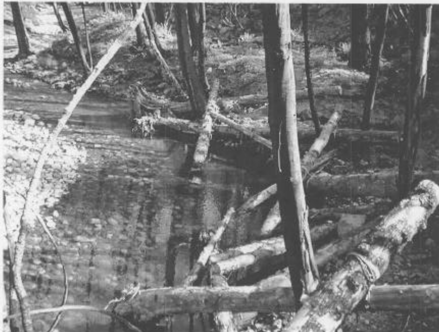
Figure 29: Completed placement of woody debris in stream
