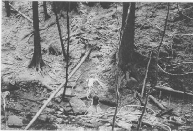
Figure 23: Hydroseeding
