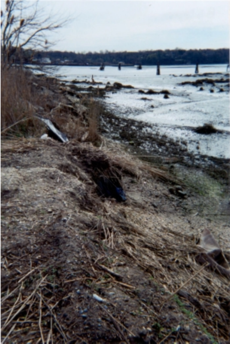
Photograph 7: The northern most shoreline of the Bar Beach Lagoon, which is adjacent to the Bar Beach parking lot. Note the sharp slope containing rubble and debris. The material that makes up the shoreline is a mixture of loosely consolidated soil and rubble/debris, which makes the shoreline moderately unstable.
