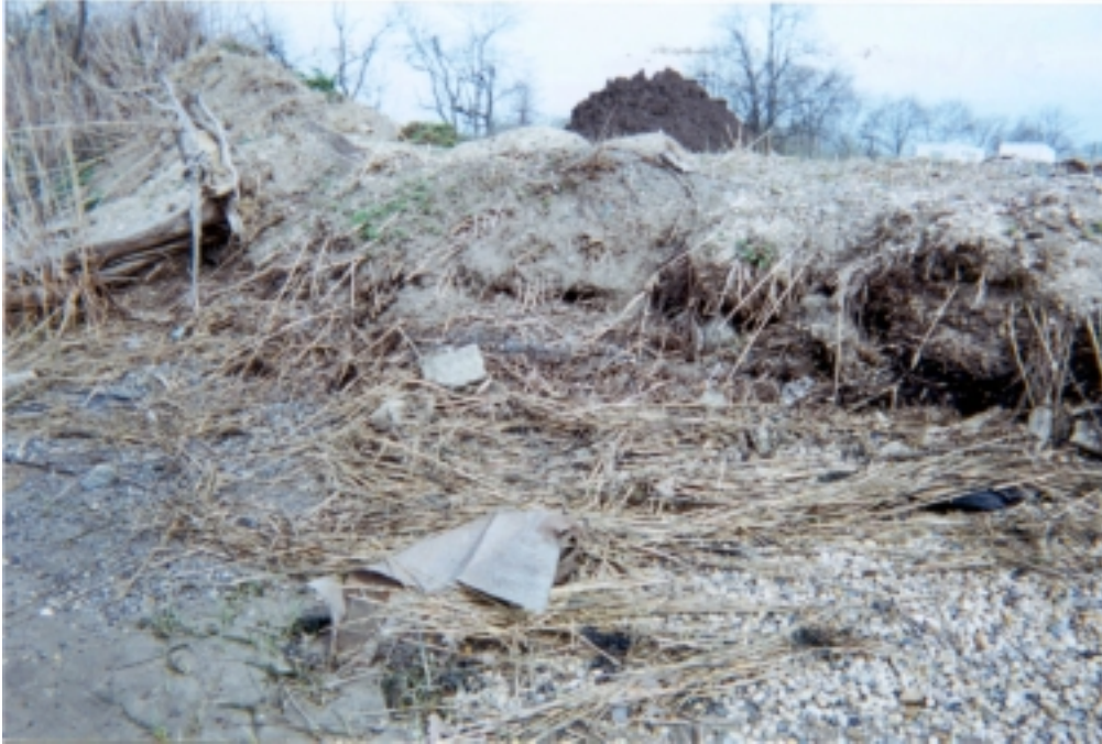
Photograph 10: Close-up of the material that makes up the shoreline. The shoreline is mostly loosely consolidated soils with a significant amount of cobble sized (and larger) rubble.
