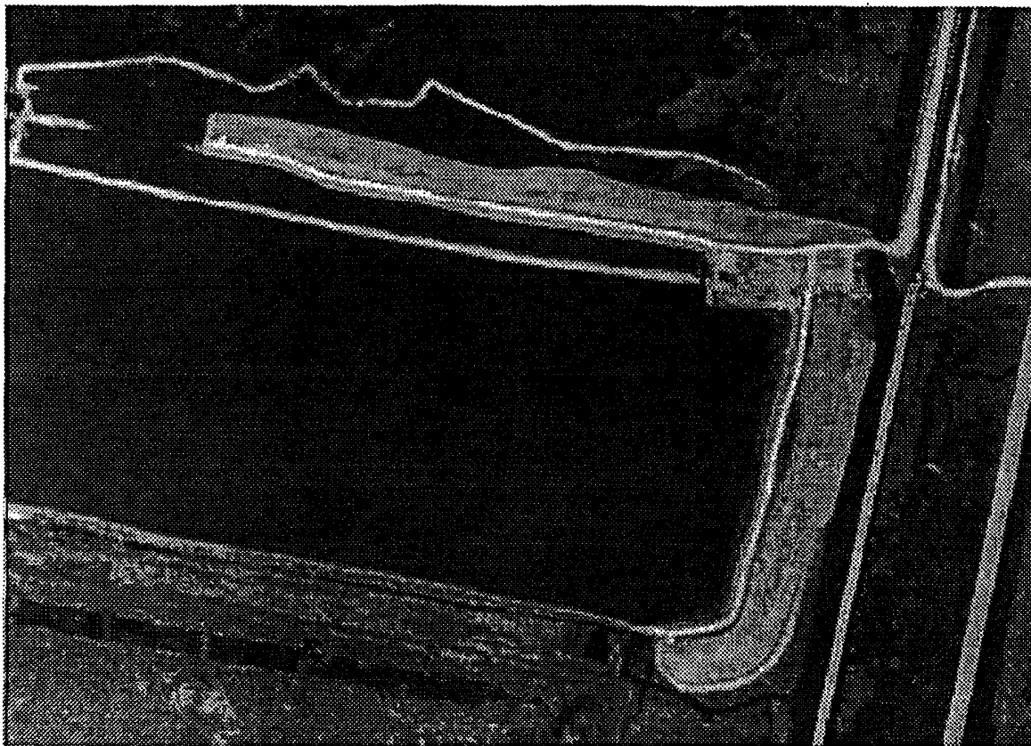
Figure 2-2. Completed remedial construction, Bailey Waste Disposal Superfund Site, Orange County, Texas.
