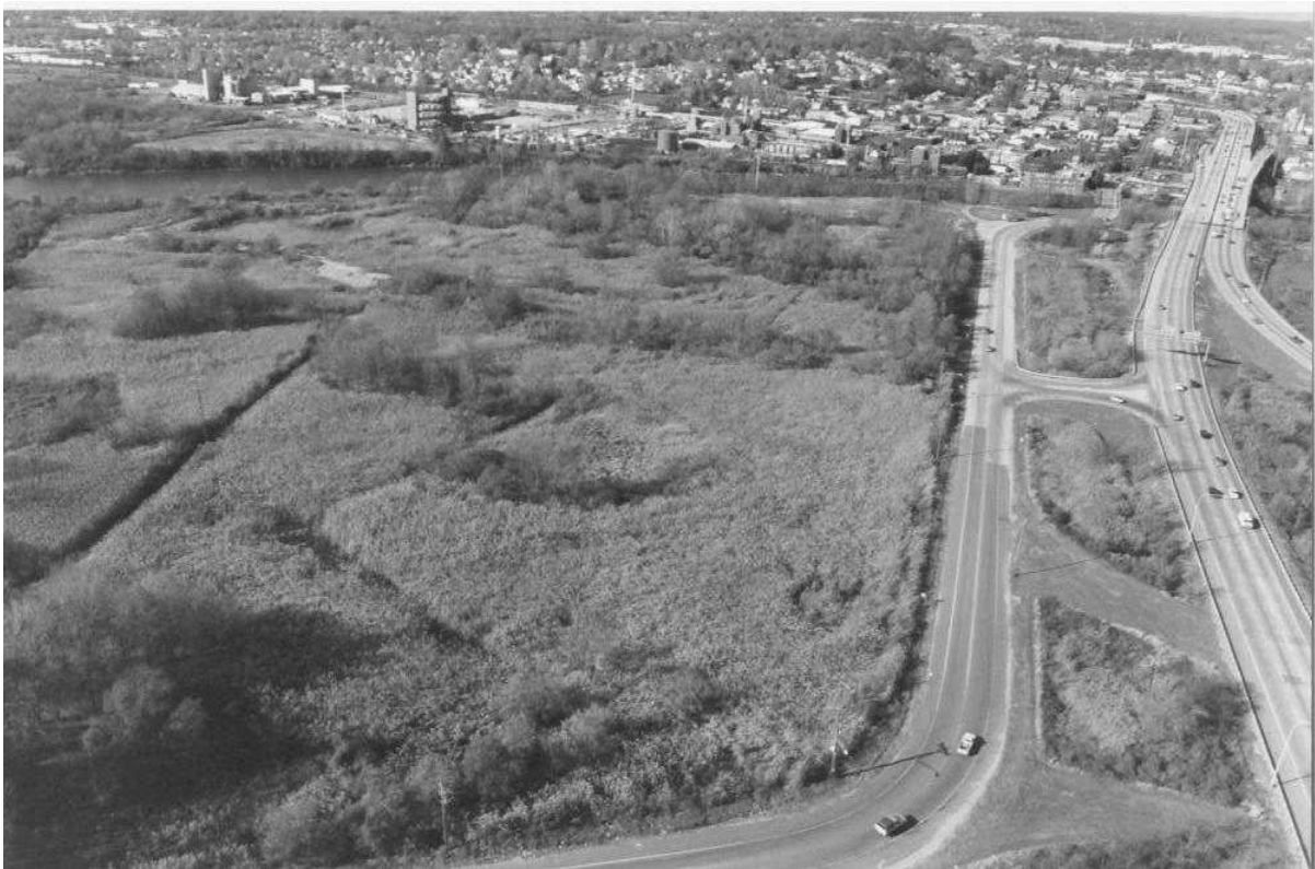
Figure 2-4 - South Wetland – Pre-remediation (looking from the S).
