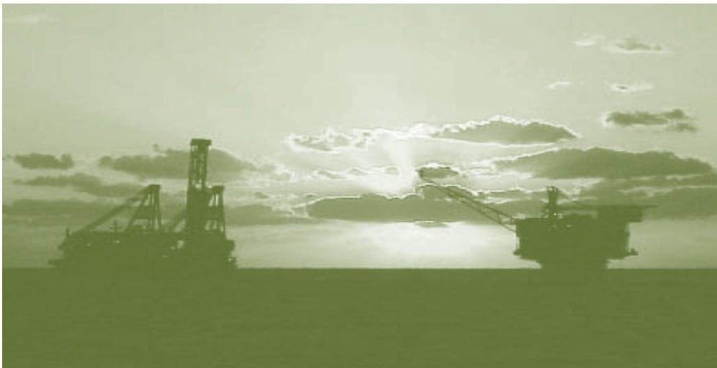
Sunset on Spar platform and construction barge in the Gulf of Mexico.
