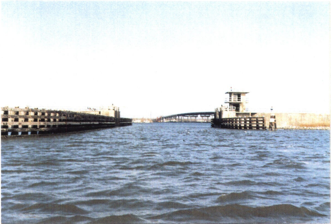
PHOTO NO. 1 - VIEW LOOKING NORTH ALONG THE CENTERLINE OF EMPIRE FLOODGATE.
