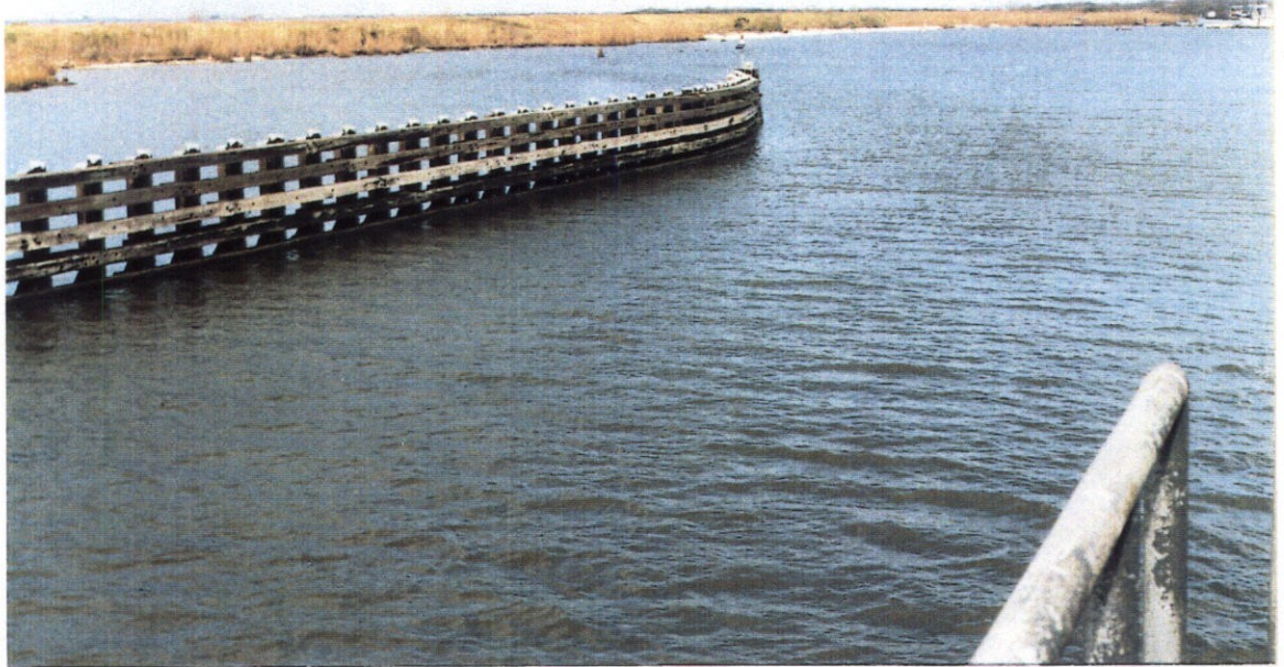
PHOTO NO. 20 - VIEW OF NORTHWEST TIMBER GUIDEWALL.
