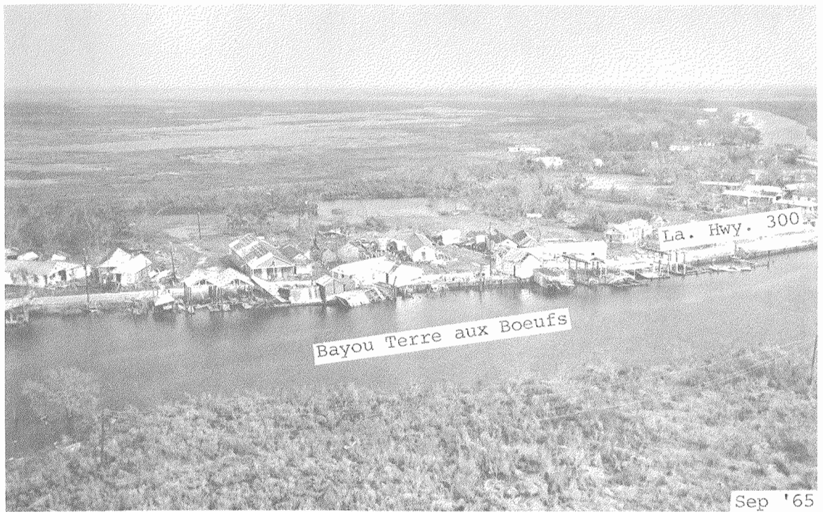
Photograph 15. Bayou Terre aux Boeufs after Hurricane "Betsy"
