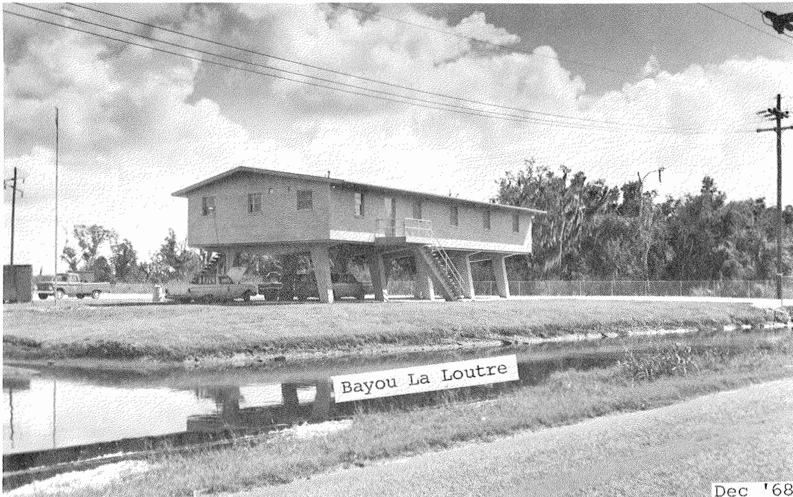
Photograph 4. Shell Oil Company office building near Yscloskey
