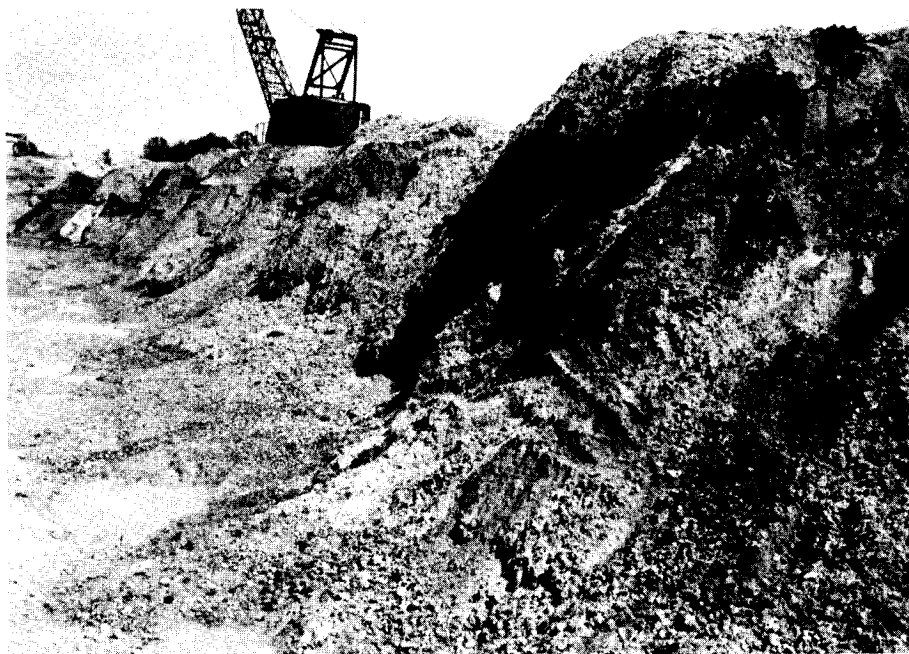
Close-Up of Working Face
