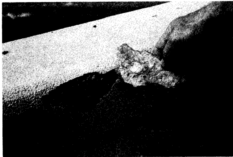
Close-Up of a Porous Chert Popout I-20 - I-220 Bypass Bridge
