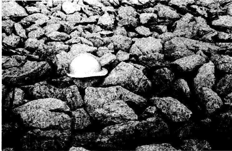
Close-Up of Bank Protection Stone Kentucky Dam, KY
