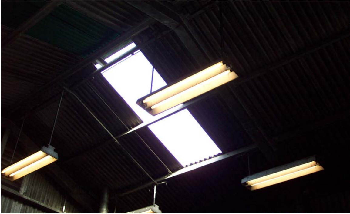
Photo 1 – Skylight panel missing.
