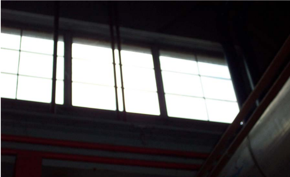
Photo 1 – 16” x 22” windows broken.
