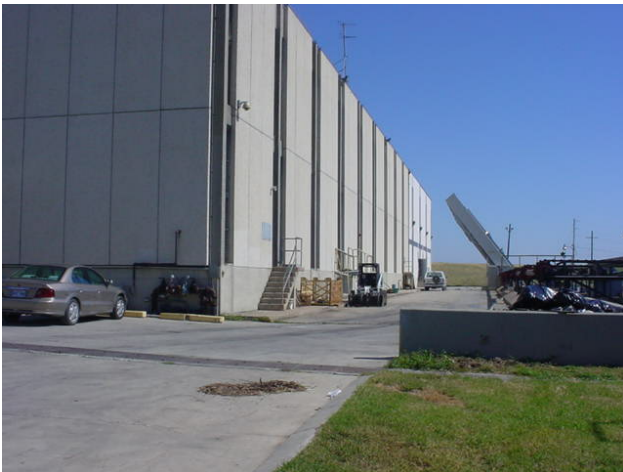
Photo No. 3 Damage Lighting
