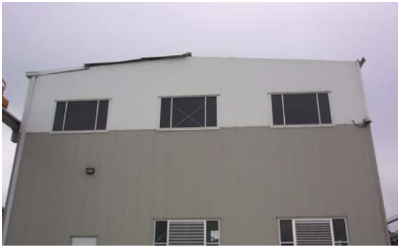
Photo 2 – Gutter and flashing damage; downspout missing. Photo No.3- GenSet controller damaged by rainwater
