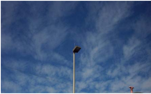
Photo No.5- Unaffected lighting pole, fixture, and air terminal
