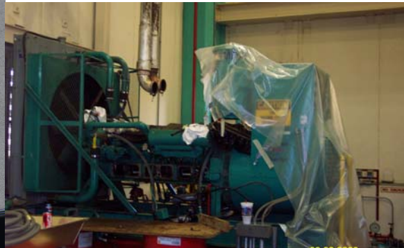
Photo No.6- GenSet Currently under repair
