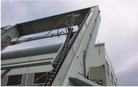
Photo 1 – Metal guard for electrical wiring in trash rack broken. Currently being repaired.
