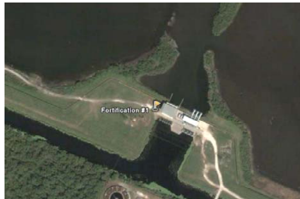
Pre-Hurricane Katrina – Aerial view of pump station
