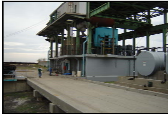
Post-Hurricane Katrina – View from the Inlet Canal
