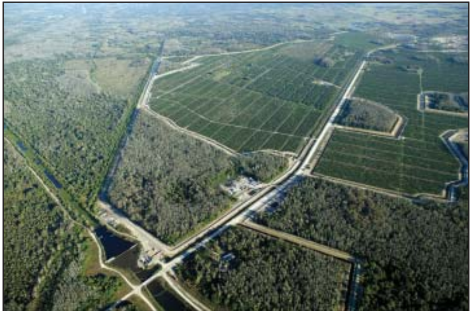
The USACE water retention area and feeder canal of the Seminole Big Cypress Water Conservation Project will enhance the quality of water in the 52,000-acre Big Cypress Reservation of the Seminole Tribe in Florida and nearby Big Cypress National Reserve and Everglades. The project will also improve wetlands by returning more natural hydroperiods. (USACE)
