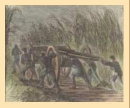
"The work was done in the following manner: The pieces, mounted on their carriages and limbered up, were moved forward on shifting runways of planks about 15 feet long, 1 foot wide, and 3 inches thick, laid end to end..."
