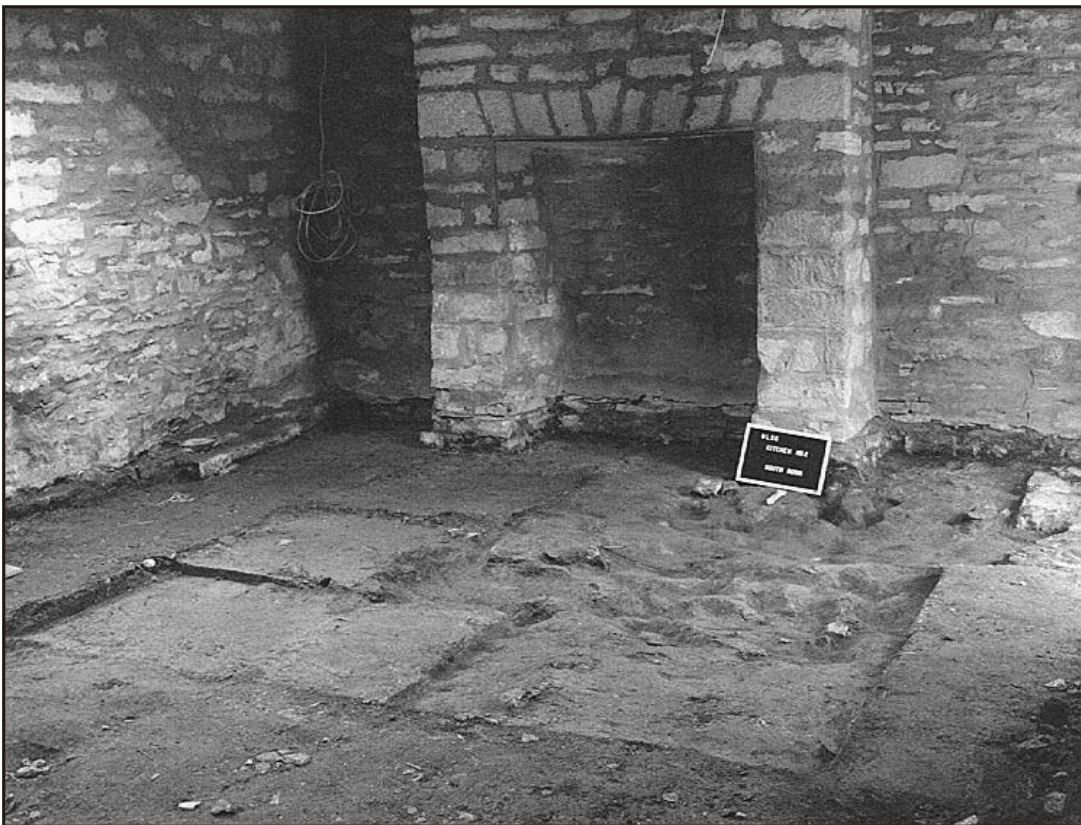
Figure 10. During 1999 the Summer Kitchen (HS-2) was excavated in preparation for its restoration; some of the excavation units and the large fireplace in the kitchen's south room are shown.
