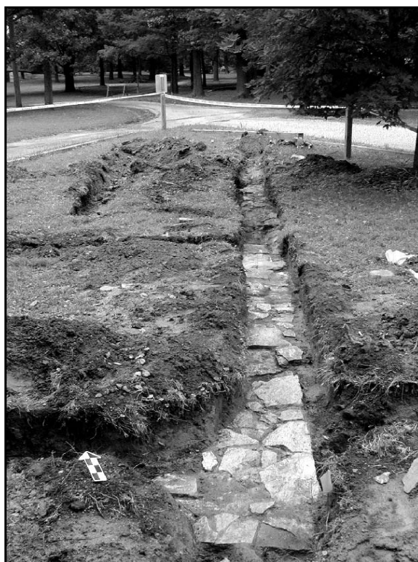
Figure 12. One feature found during the 2000 shovel testing and further extensively tested is a massive stone foundation that is probably associated with an 1818-era barn.
