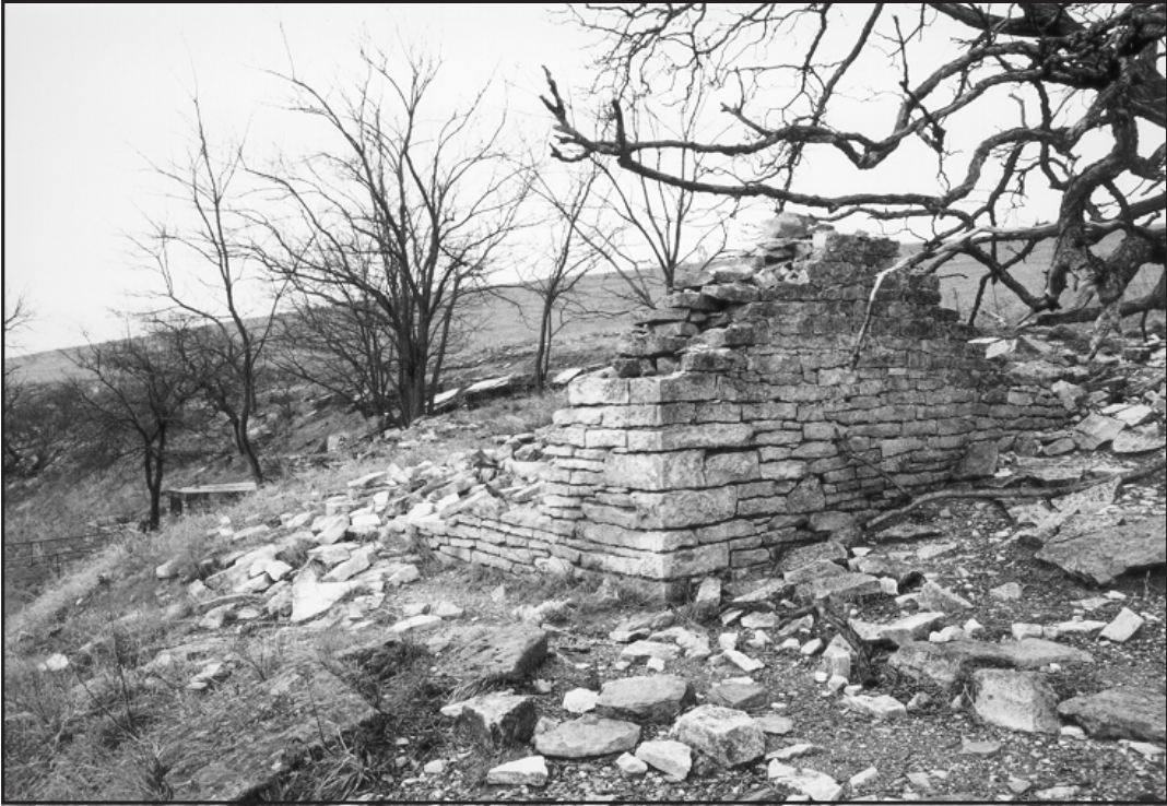
Figure 15. 14CS111, Tallgrass Prairie National Preserve. Northeast corner of standing structure. View to the southwest.
