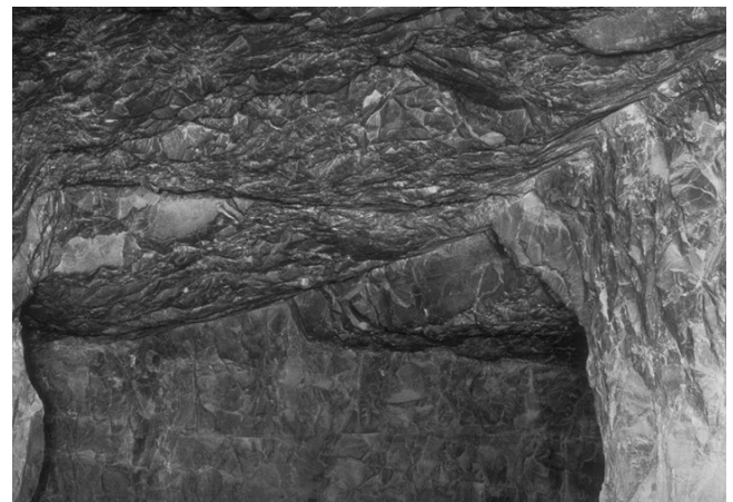
Figure 7. Unstable roof associated with typical low-angle thrust faults.
